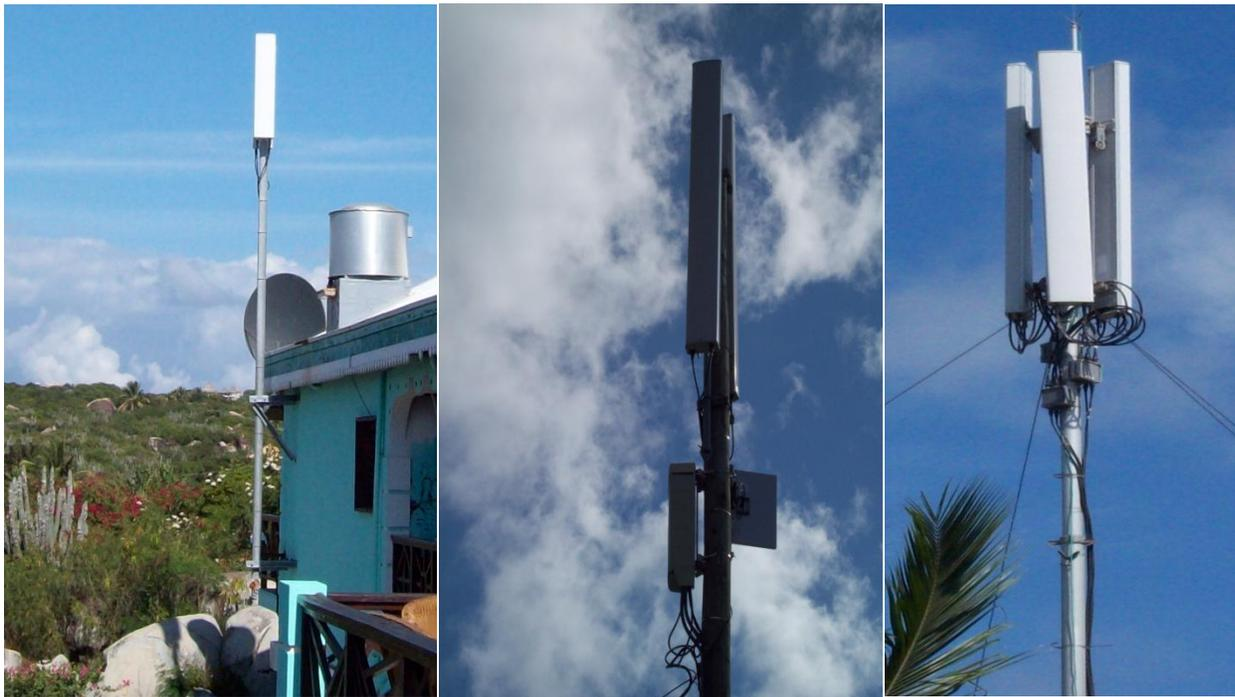
**Figure 27 - Examples of Sector-based Installations at Cell Sites**
